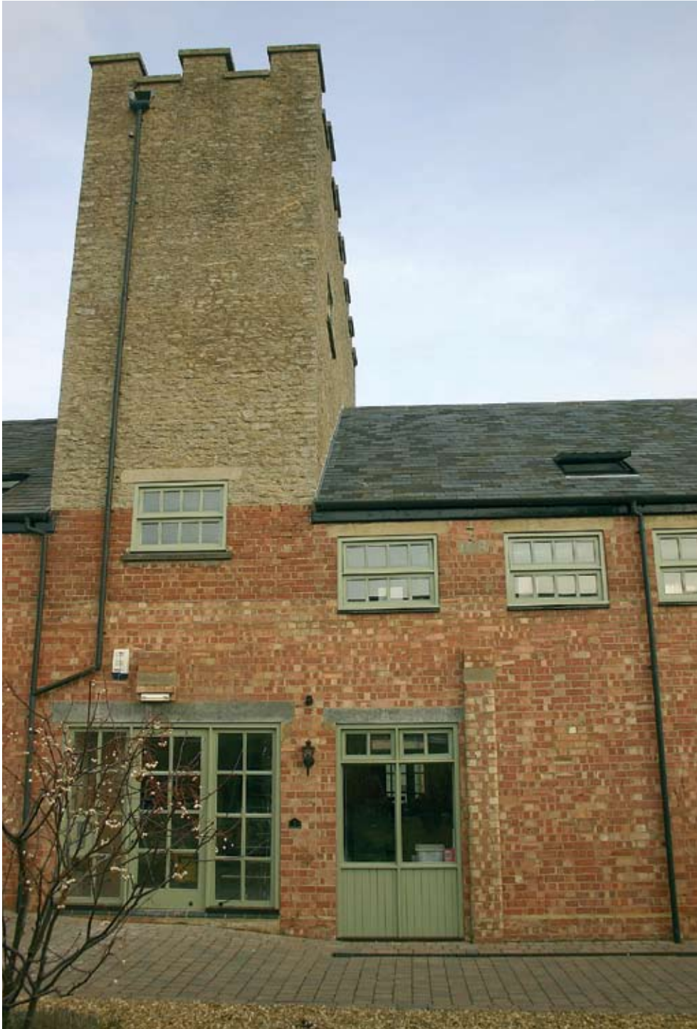
Exterior from central courtyard, showing original water tower
